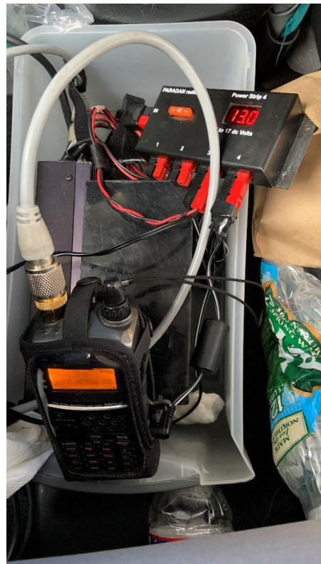
Amp, Battery, radio and my power splitter/volt meter in plastic box in back floorboard.
